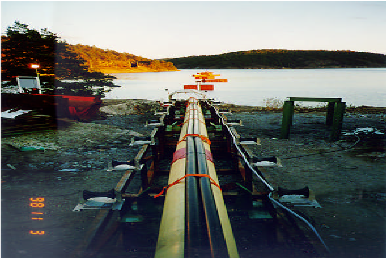
Figure11-Installation of field test flowline section (380m long)
