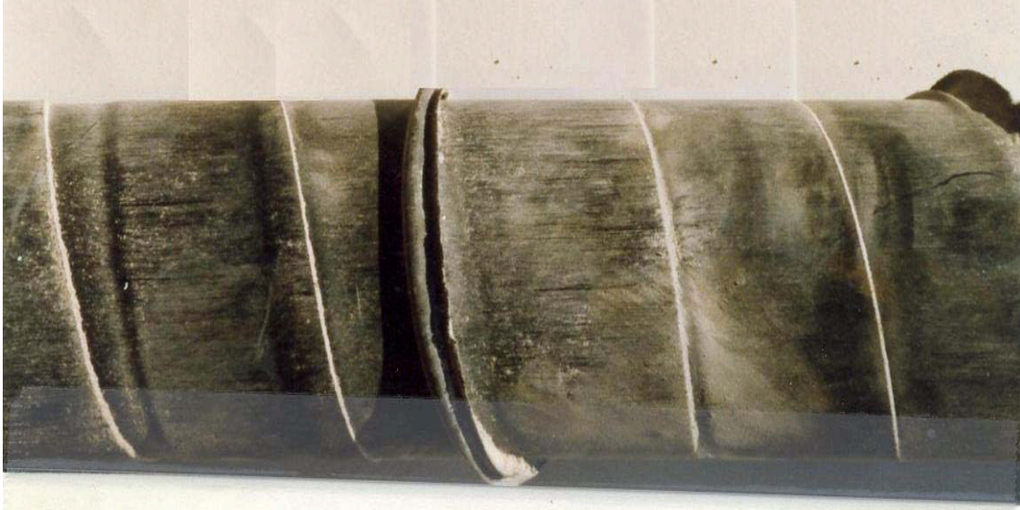
FIGURE 11 – Failure at Weak Overlaps.
