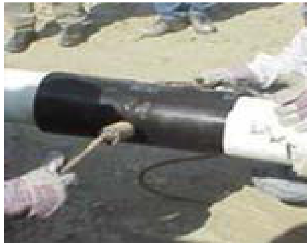
FIGURE 5 – Heat-Shrinkable Sleeve
