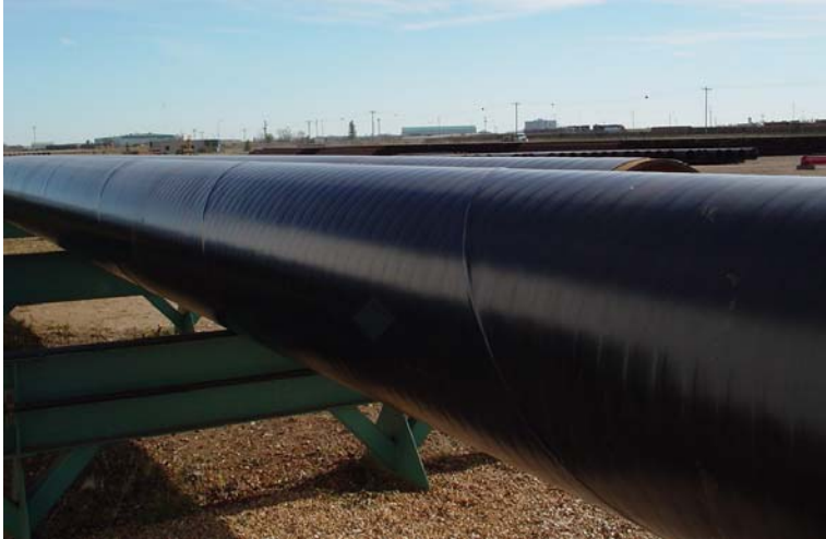
(a) Side-Wrapped GSPE on Spiral Weld Pipe (30")
