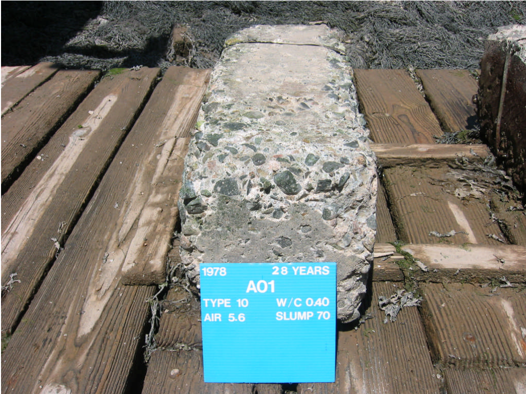
Figure 3. Phase I: 11.4% C 3 A, 0.4 water/cement ratio (Courtesy of CANMET)
