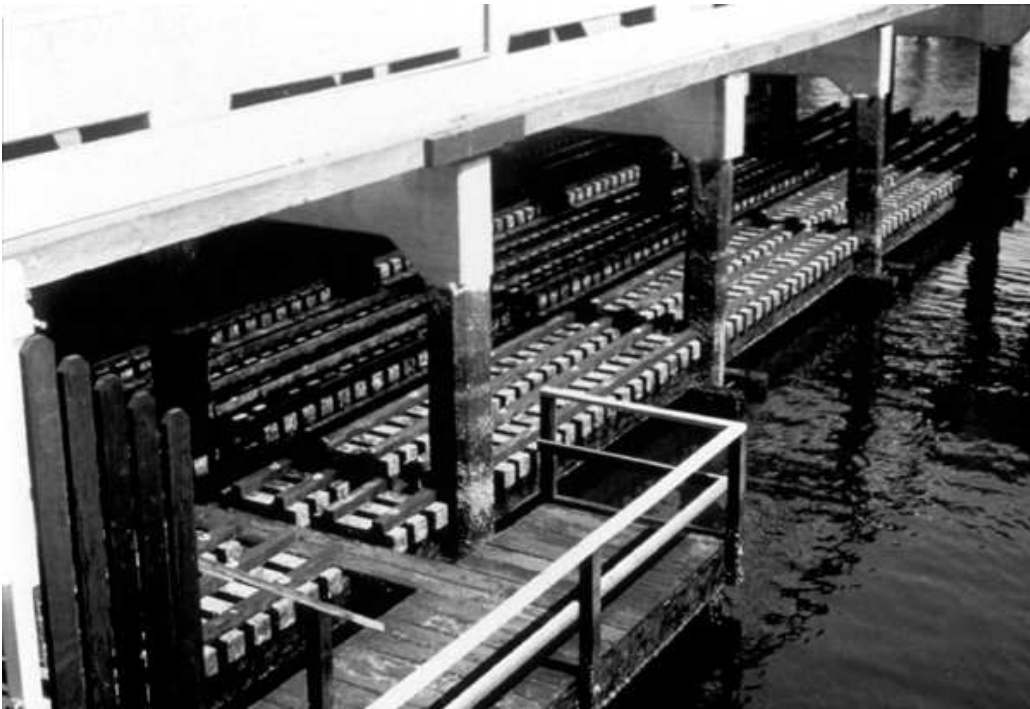
Figure 6. PCA Long-time Durability Test Site in Los Angeles Harbour. (Courtesy of the Portland Cement Association)
