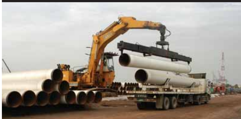
▼ 3LPP Coated Pipes Destined for Qatargas 3 & 4
