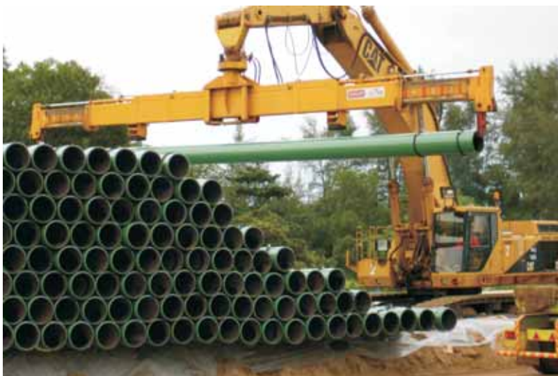
▲ FBE coated pipes protected for the Gumusut-Kakap Deepwater Project
