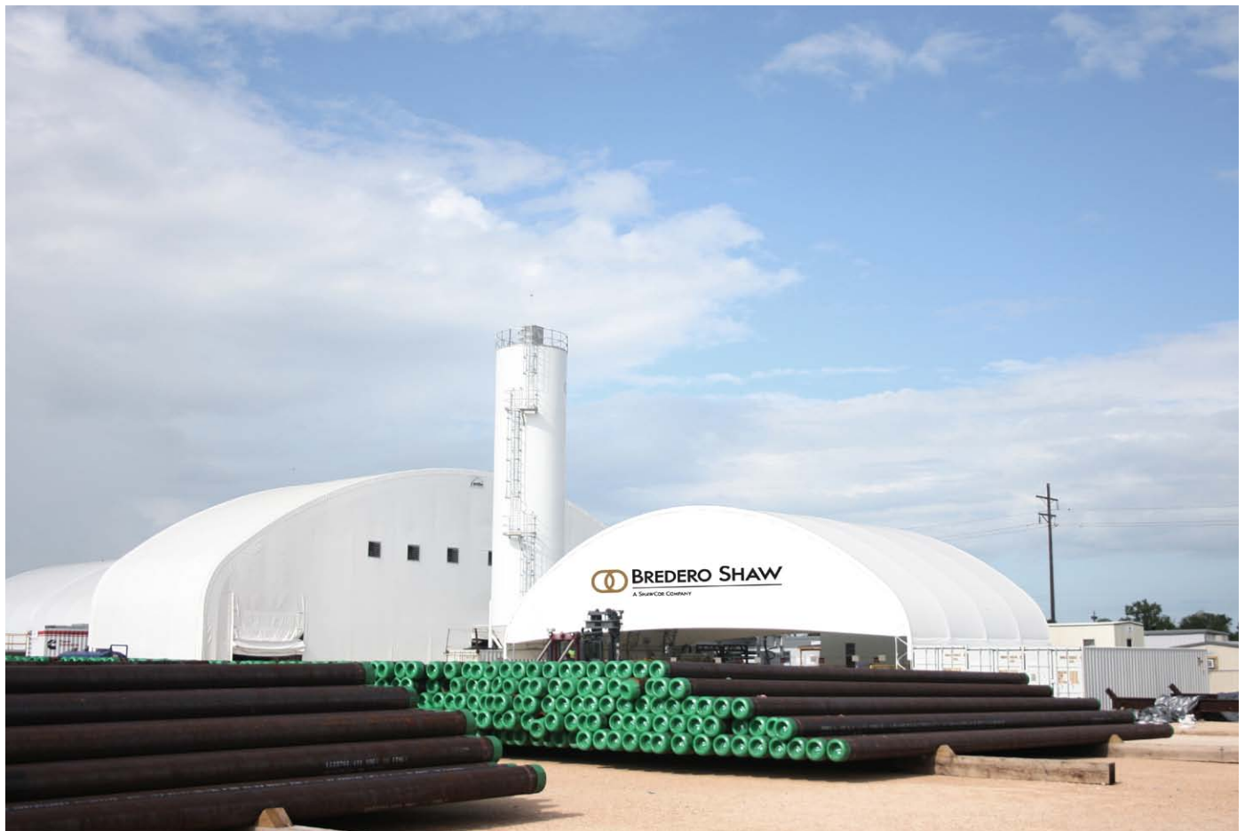
Figure 2. Bredero Shaw's new Brigden modular facility.
